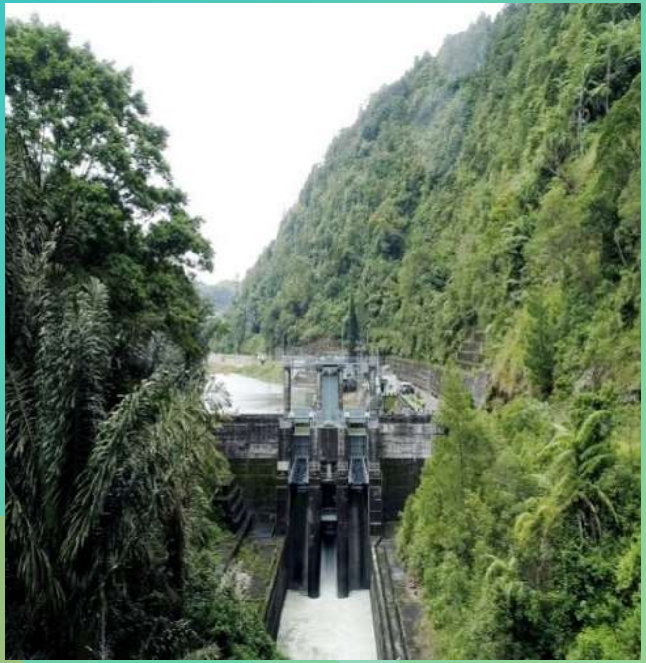
PLTA Asahan with capacity of 603 megawatts (MW)
